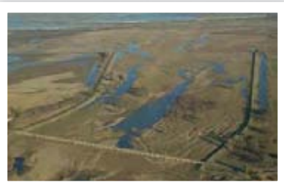
The Colusa Weir, its training levees, and sediment basin are SPFC facilities
