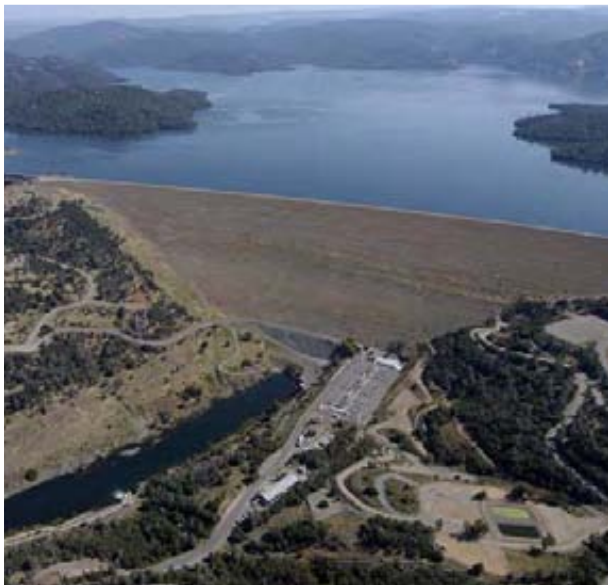
Oroville Dam is part of the SPFC
