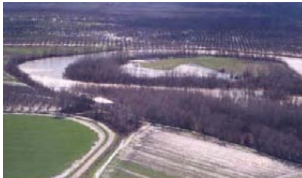
The SPFC relies on the Three B's Natural Overflow Area to protect downstream levees on the Sacramento River
