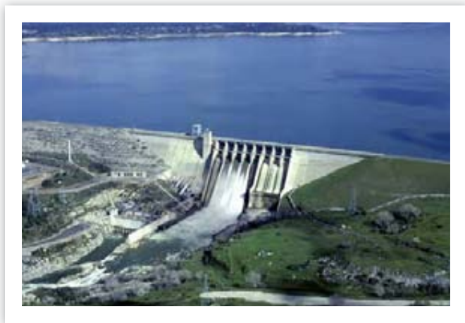
Construction of the American River Watershed, Folsom Dam Raise Project is underway
