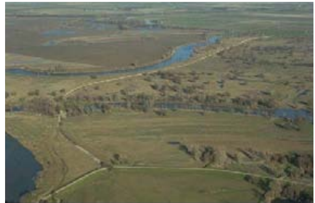
Fremont Weir (photo courtesy of NOAA)
