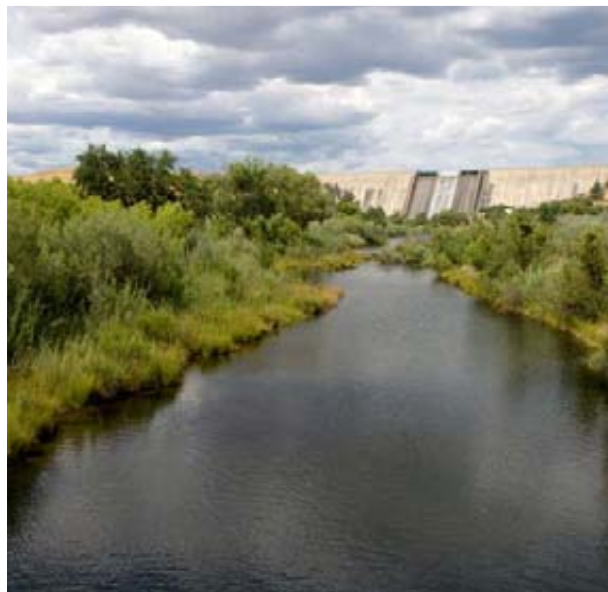
Friant Dam is operated for multiple purposes, including flood management (photo courtesy of Anne Canright)
