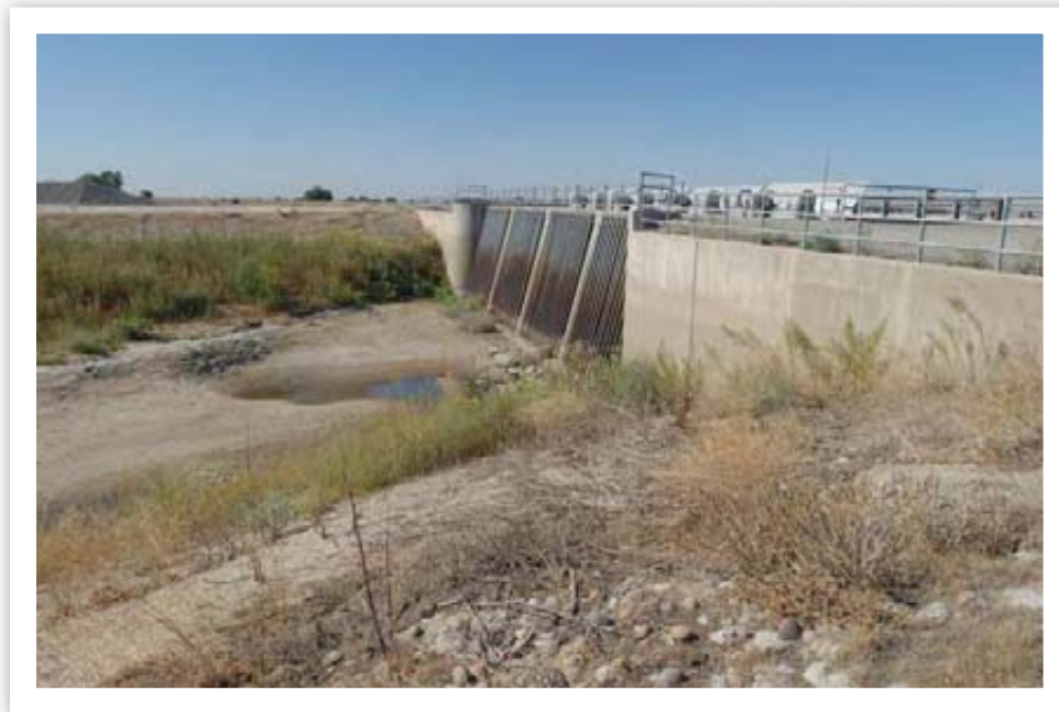
The Chowchilla Canal Bypass Control Structure is an SPFC facility
