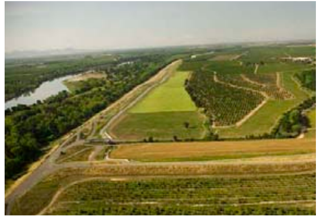
The Bear River Setback Levee was constructed under the Early Implementation Program
