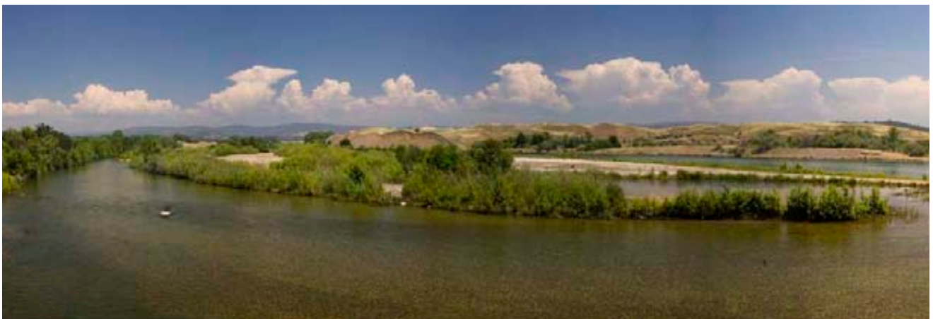
SPFC facilities include right-and-left bank levees on the Yuba River
