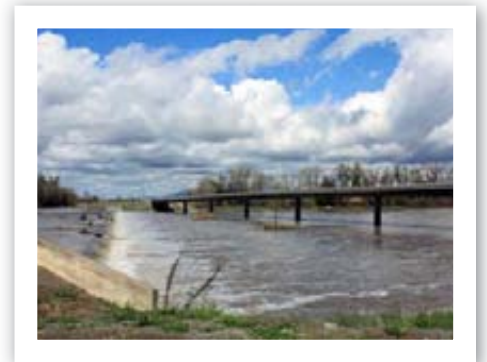
Tisdale Weir spills into the Sutter Bypass (photo courtesy of Sutter County)
