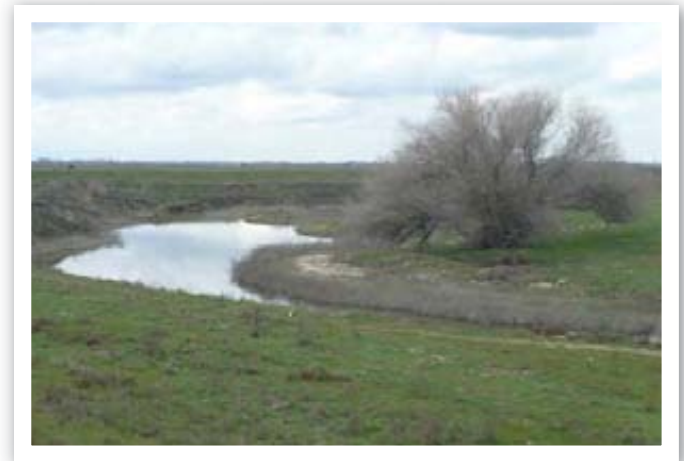
Eastside Bypass levees are maintained by Lower San Joaquin Levee District
