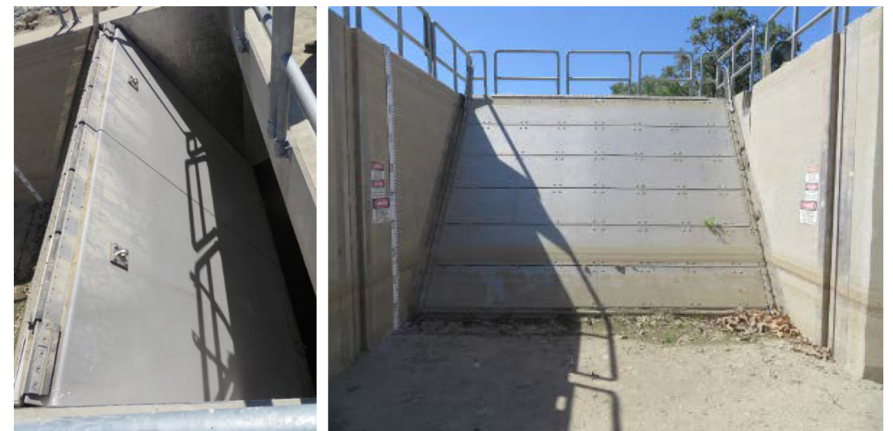
(Left) Fremont Weir front-side cover plate (covering stiffening ribs) (Right) Fremont Weir back-shield plate, showing top hinge.
