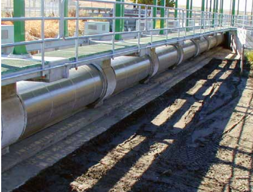
4871 Figure 10-8. Medium-sized rotary drum screen at the Burlingame Diversion located on the 4872 Walla Walla River near Walla Walla, Washington
