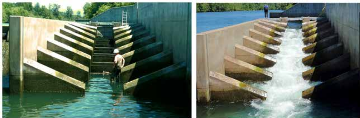
1832 1833 Figure 5-10. Pool and chute ladder dewatered (at left) and watered (at right)
