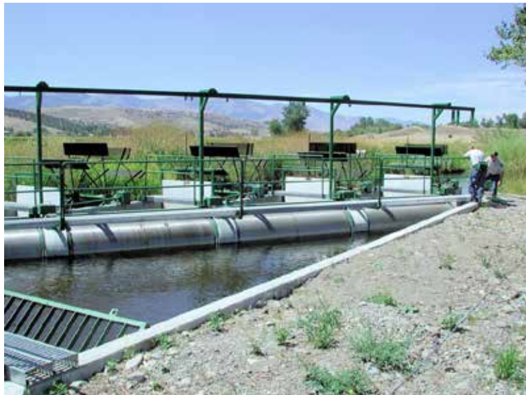
4874 Figure 10-9. Rotary drum screens installed in a water diversion canal and operated (i.e., 4875 powered) by paddle wheels
