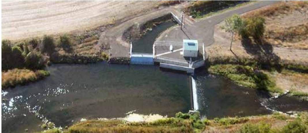
4603 4604 Figure 10-1. Aerial view of the Garden City-Lowden 2 water diversion on Walla Walla River 4605 near Touchet, Washington
