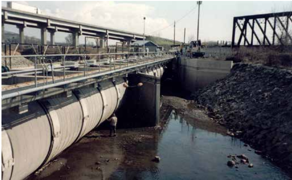
4865 4866 Figure 10-7. Large-sized rotary drum screen at the Sunnyside Canal located on the 4867 Yakima River near Yakima, Washington 4868 (Note: The person standing upstream of a drum and an intermediate bypass entrance. Water flow direction is from 4869 the foreground to the background of the photograph.)
