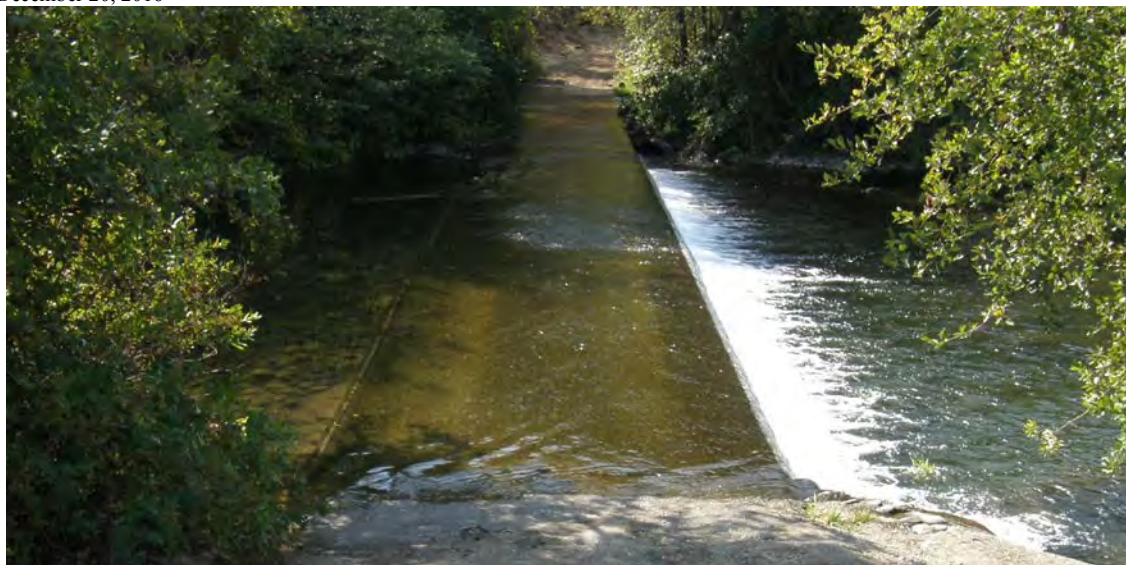
Figure 18 Antelope Creek lower slab pre 2014 high flows
