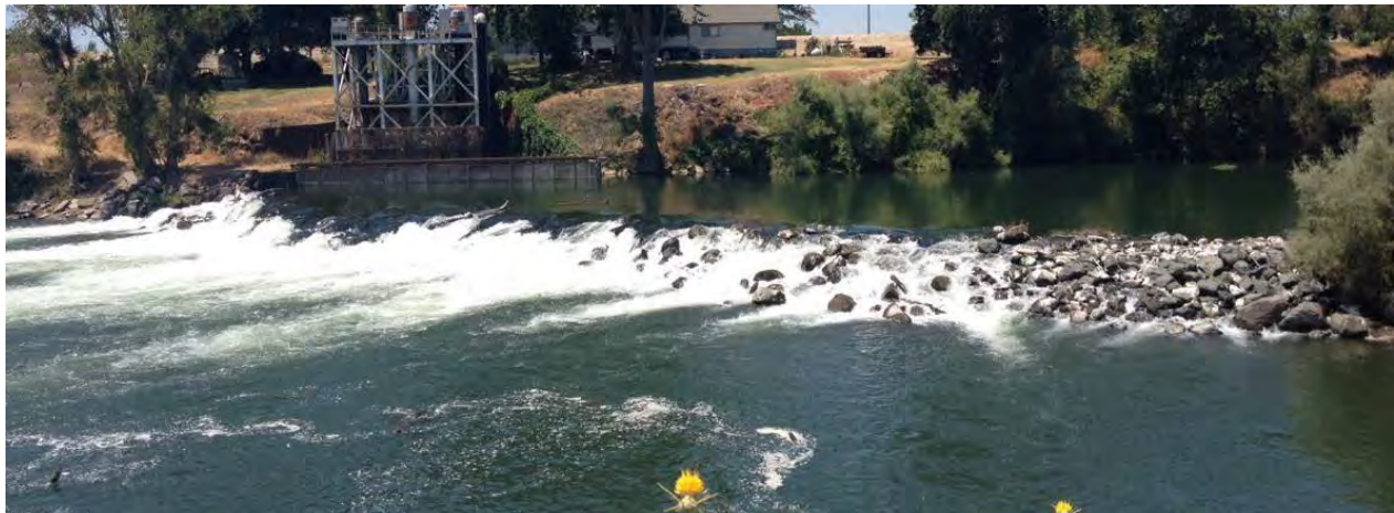
Figure 2 Sunset Pumps weir
