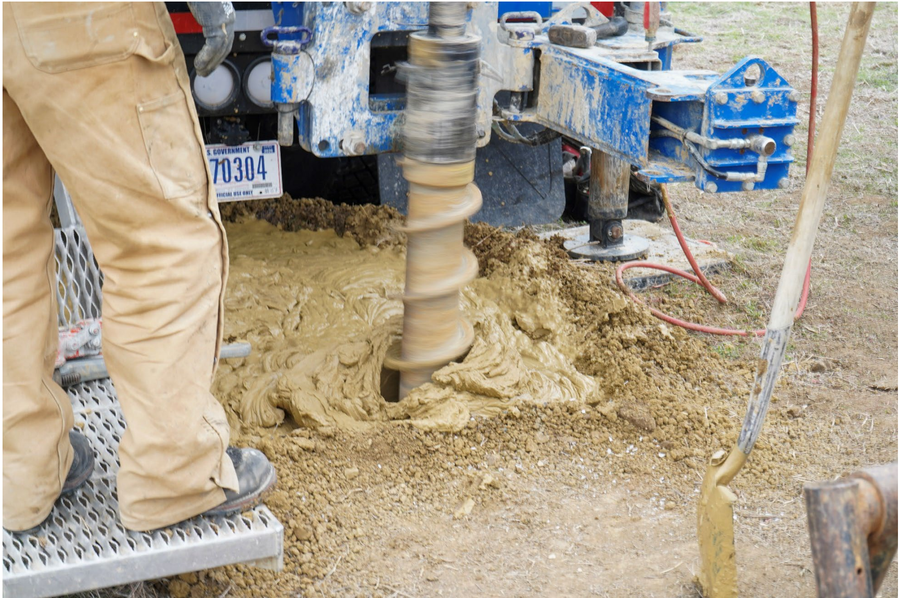
Photo 4 – Representative photo of rotary auger boring.
