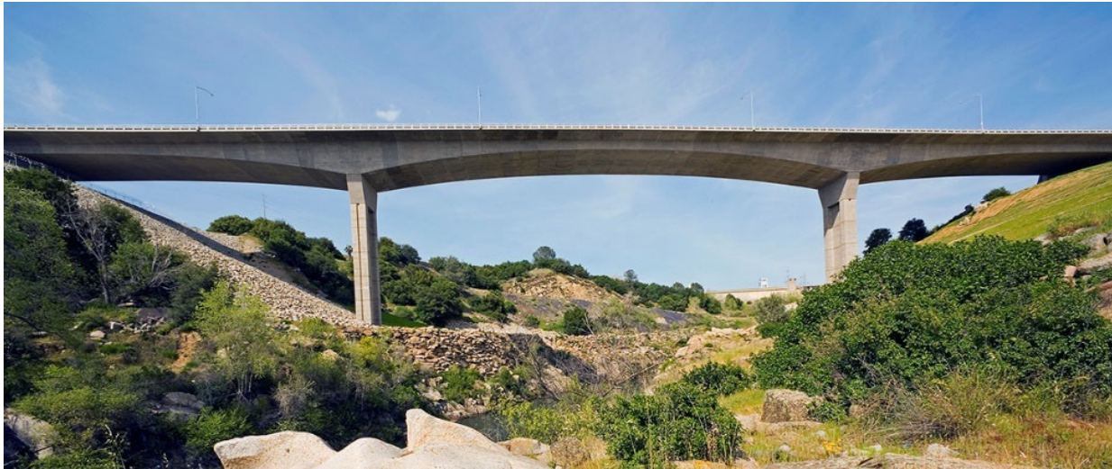
Figure 3-5 – CIP Segmental Box Girder, Folsom Dam Bridge
