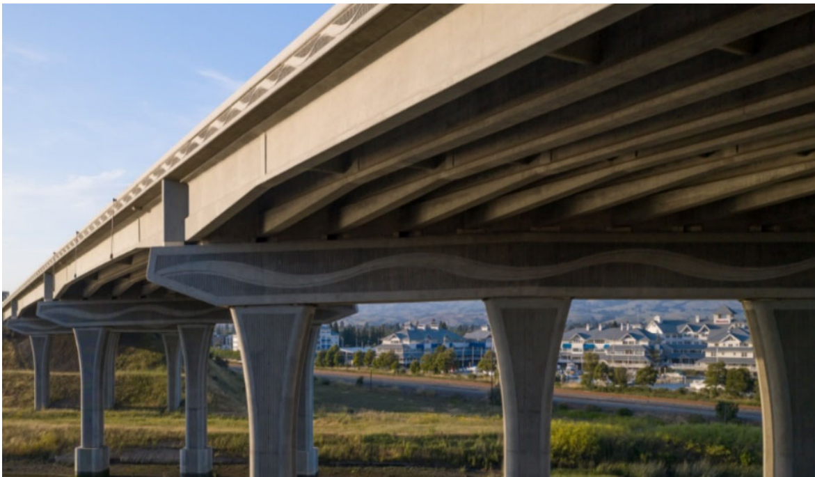
Figure 3-4 – Precast Spliced Girder, US 101 Petaluma River Bridge
