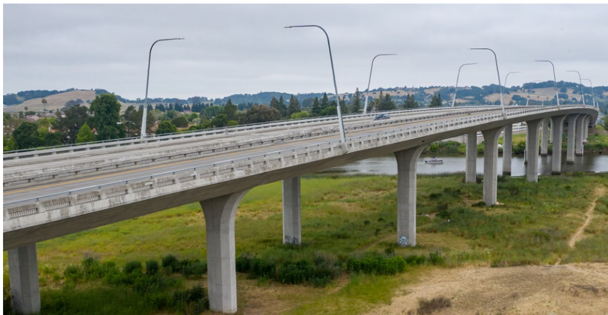
Figure 3-3 – CIP P/S Box Girder Bridge, West Imola Avenue (SR 121) Over Napa River
