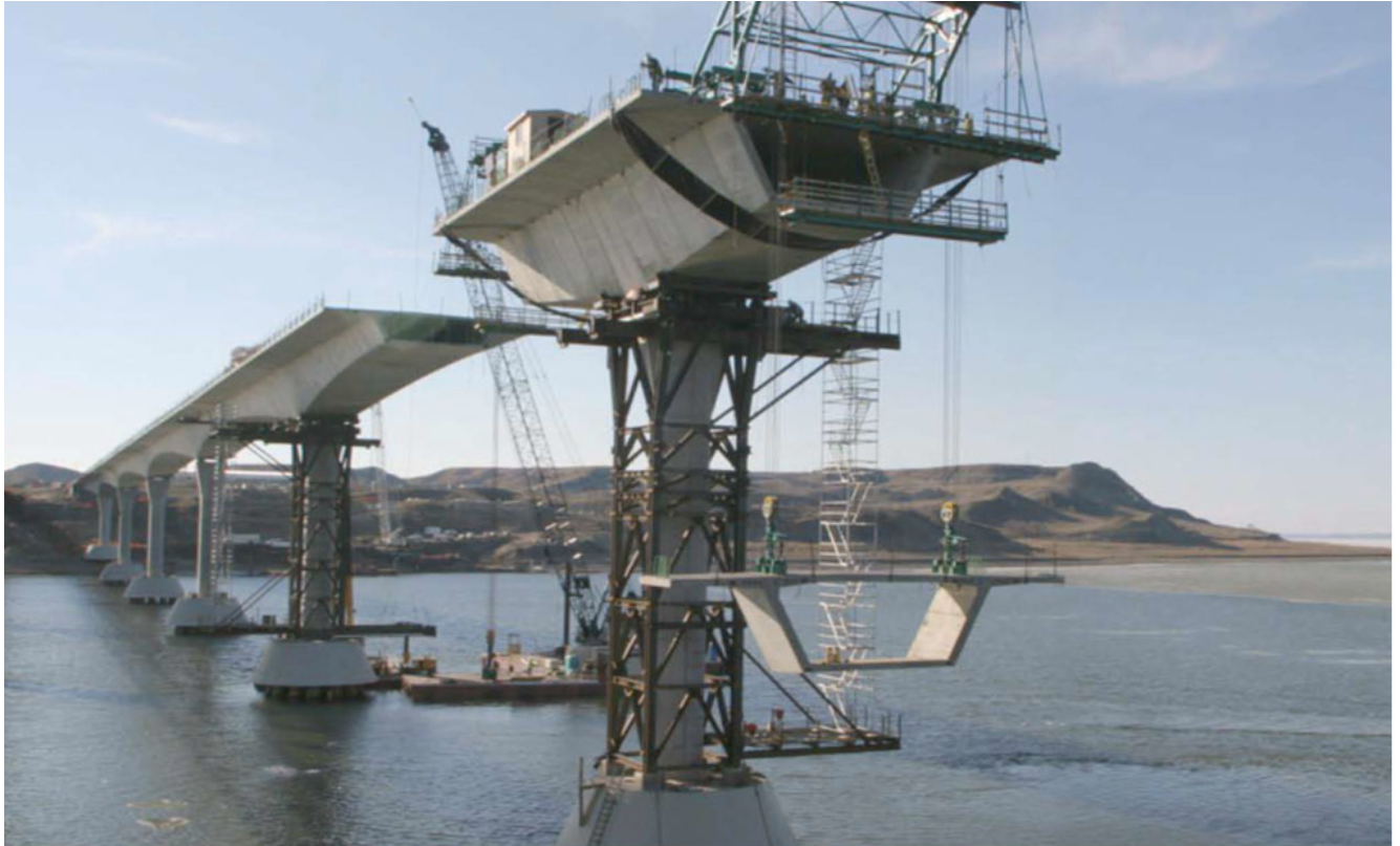
Figure 3-6 – Typical Erection of Precast Elements
