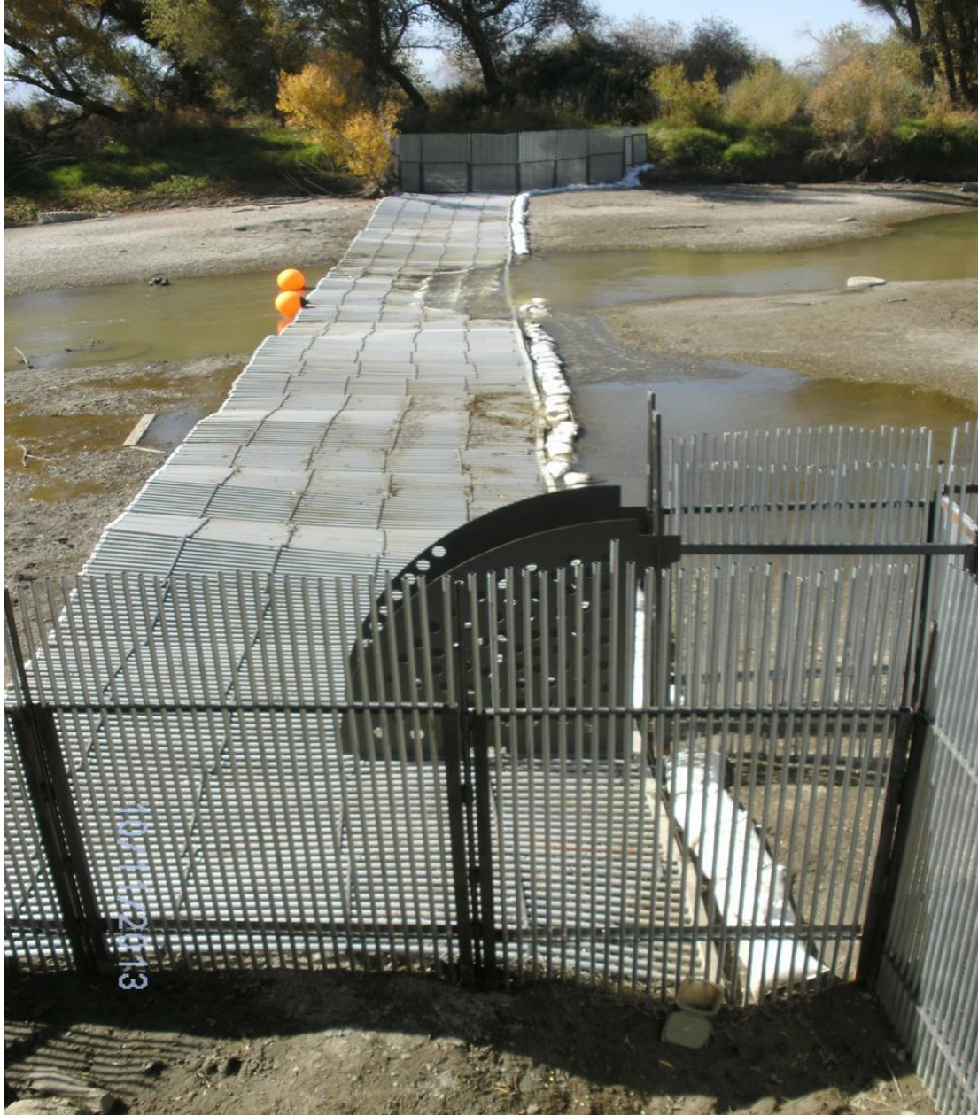
Figure 6. Photo of the Colusa Basin Drain weir and trap entrance.
