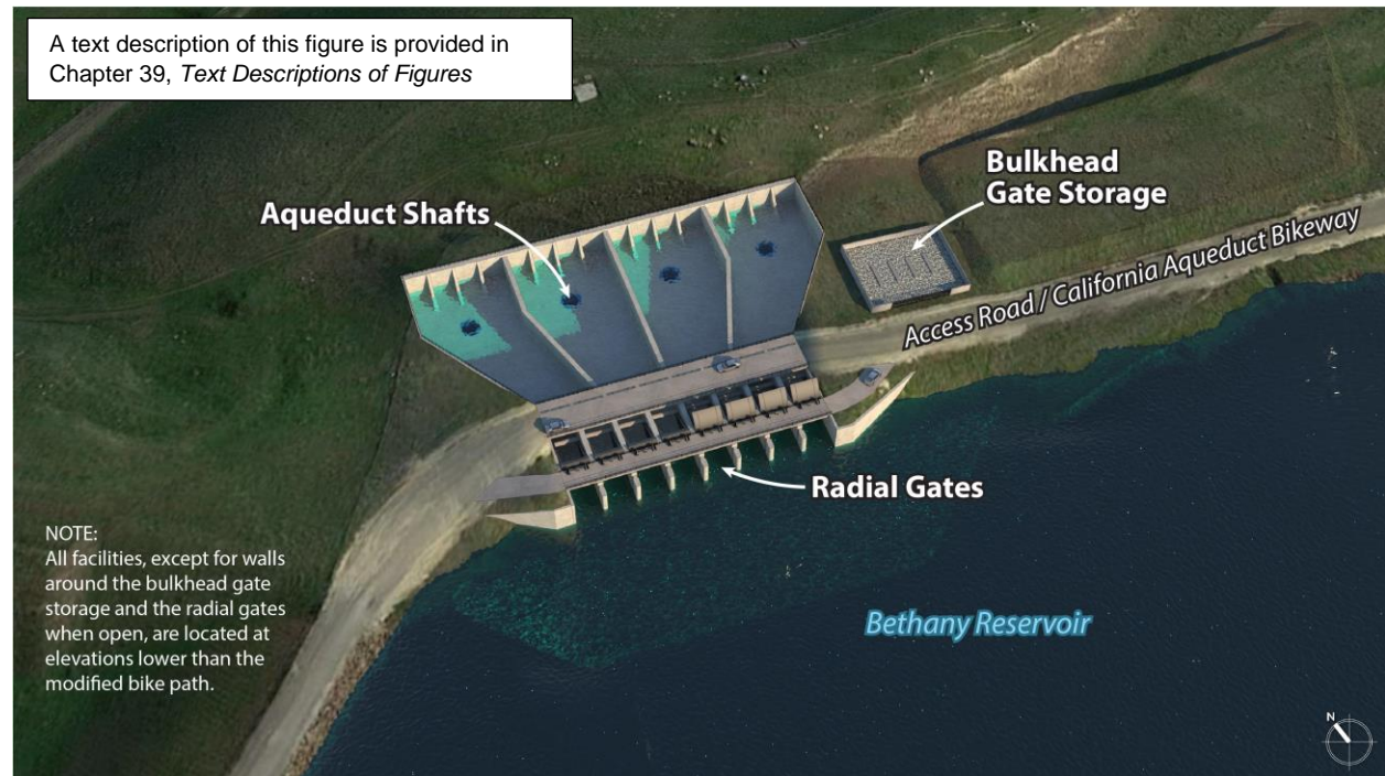
4 5 Figure 3-34. Bethany Reservoir Discharge Structure
