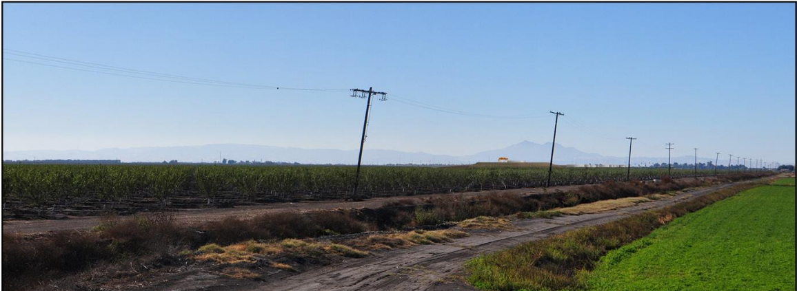
Rendered View During Construction
