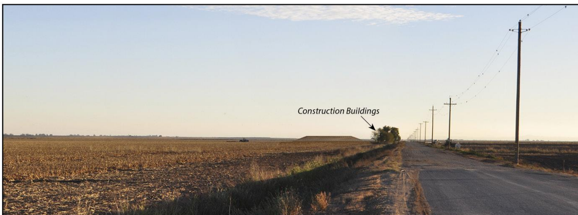
Rendered View During Construction
