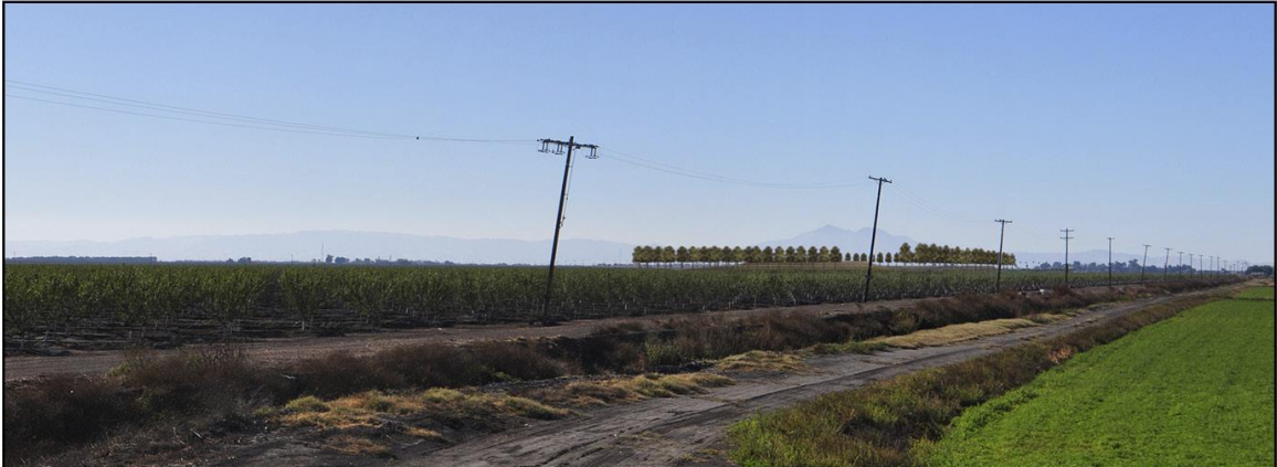
Rendered View After Construction (Note: Assumes removal of construction-related buildings and gantry crane in work area.)
