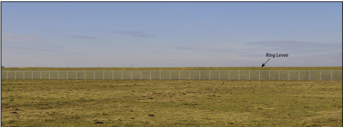
Rendered View During Construction
