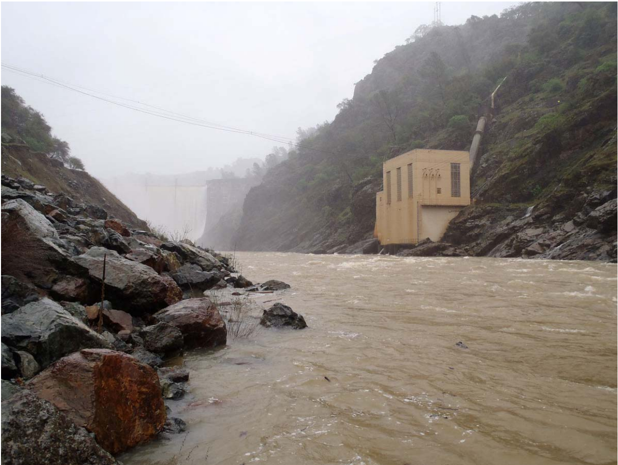
Figure 3.3-4. Yuba River below Narrows No. 1 Powerhouse on March 16, 2012. The powerhouse is on river right and Englebright Reservoir, which is spilling, is in the background.
