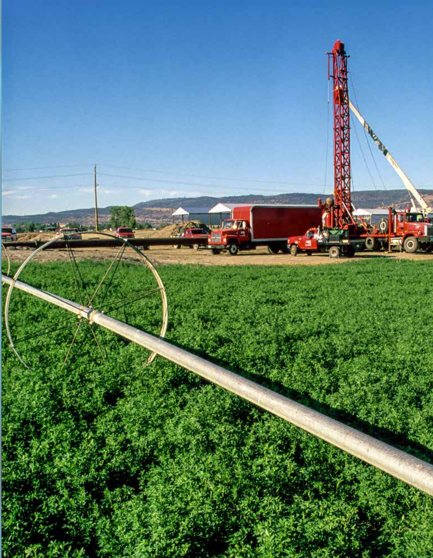
Well drilling near Tule Lake
