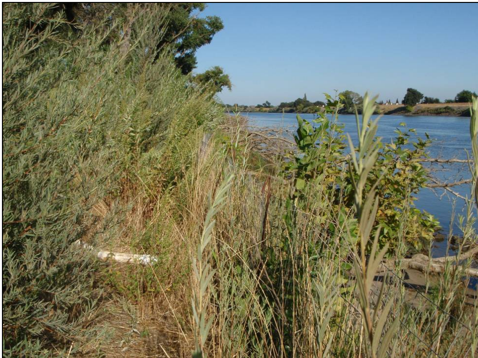
Site 43.7R, Photo-point 4. Repair site with 10:1 slope design. Note that a large portion of the installed instream woody material is above the water level. Also note the rapid development of woody riparian vegetation. Photo taken August 2009.
