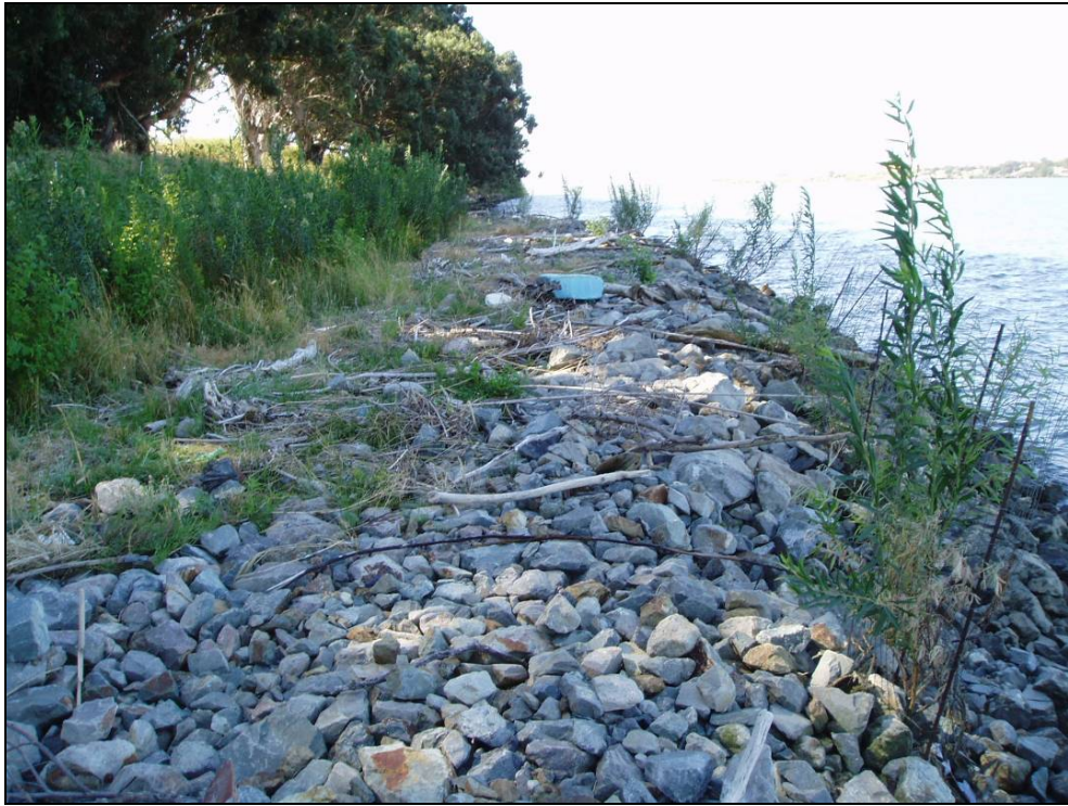
Site 12.5L, Photo-point 2. Repair site with bench design. Photo taken August 2008.
