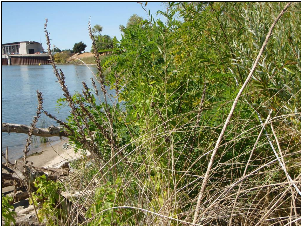
Site 47.0L, Photo-point 2. Repair site with 10:1 slope design. Photo taken August 2009.
