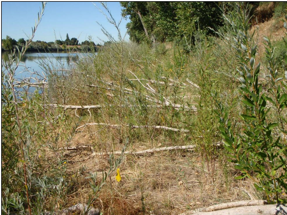
Site 44.7R, Photo-point 4. Repair site with 10:1 slope design. Note that a large portion of the installed instream woody material is above the water level. Also note the continued development of the riparian plantings. Photo taken August 2009.
