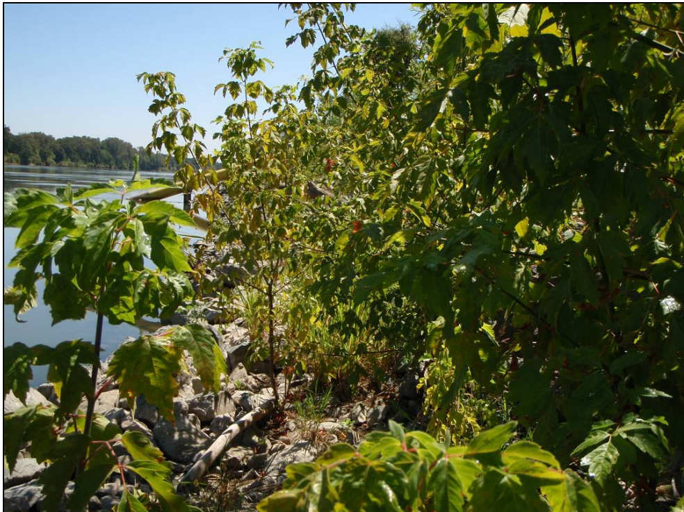
Site 69.9R, Photo-point 1. Repair site with a no bench design. Note the rapid development of riparian vegetation. Photo taken August 2009.
