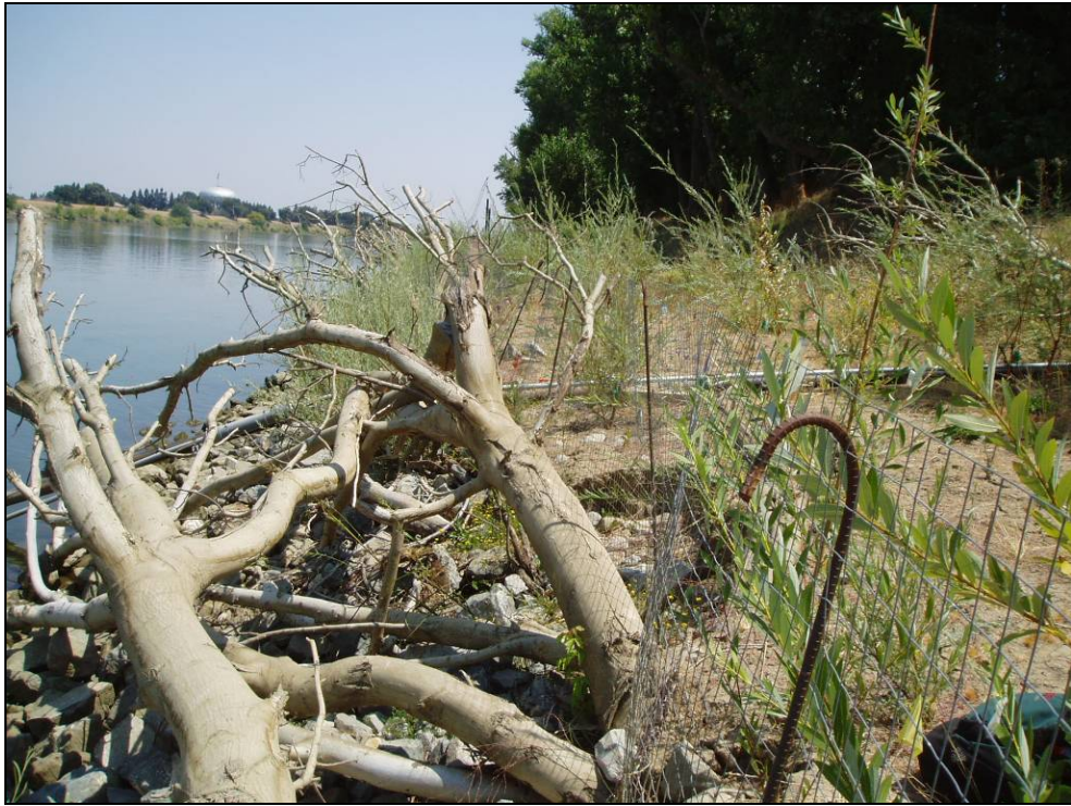
Site 47.9R, Photo-point 1. Repair site with 10:1 slope design. Photo taken August 2008.
