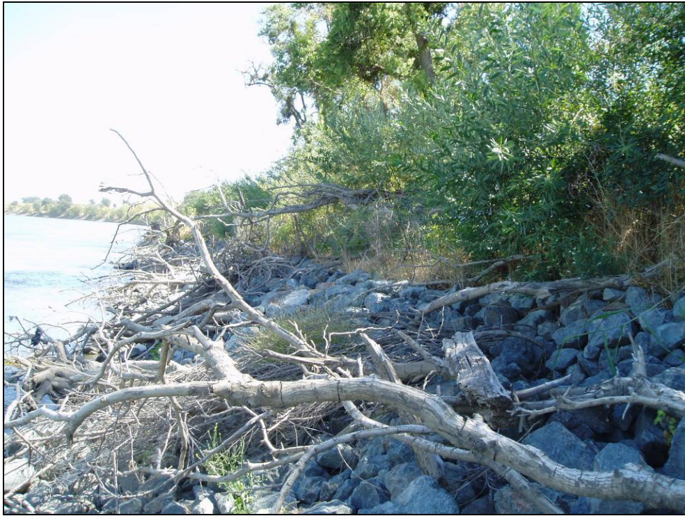
Site 85.6R, Photo-point 1. Repair site with a no bench design. Photo taken August 2008.
