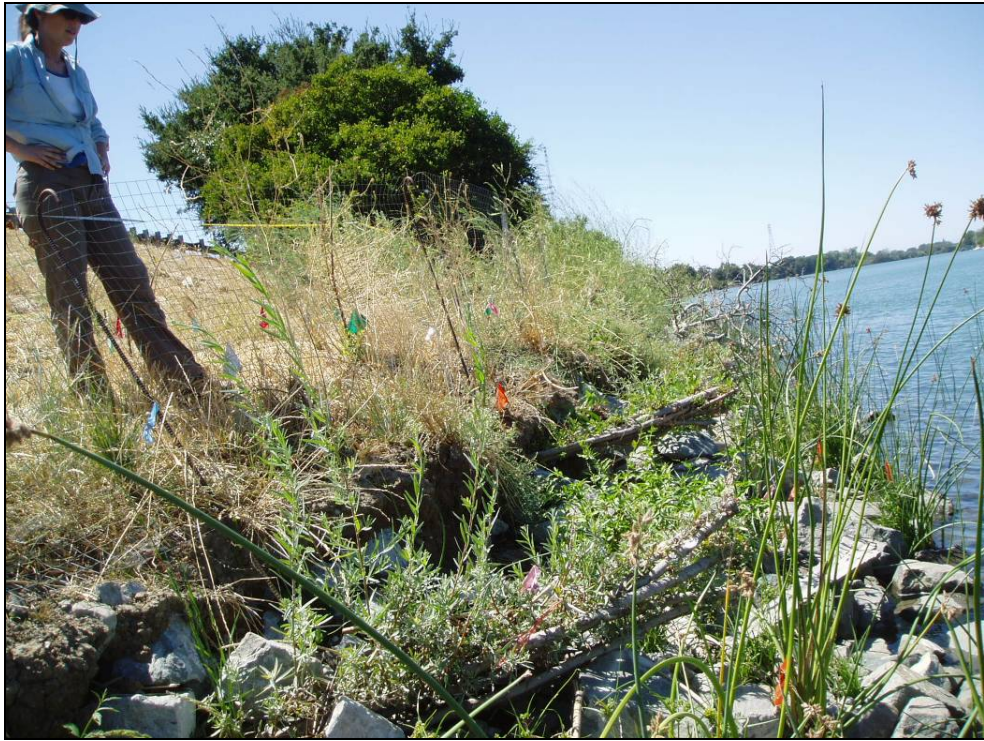
Site 16.9L, Photo-point 1. Repair site with 10:1 slope design. Photo taken August 2008.
