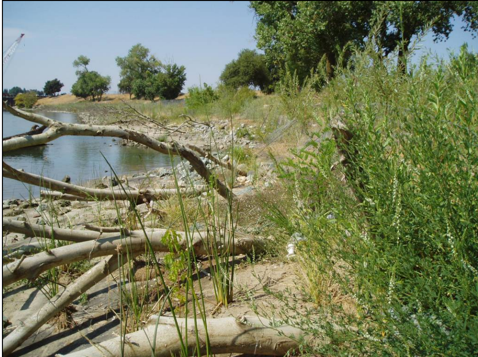
Site 47.0L, Photo-point 2. Repair site with 10:1 slope design. Photo taken August 2008.
