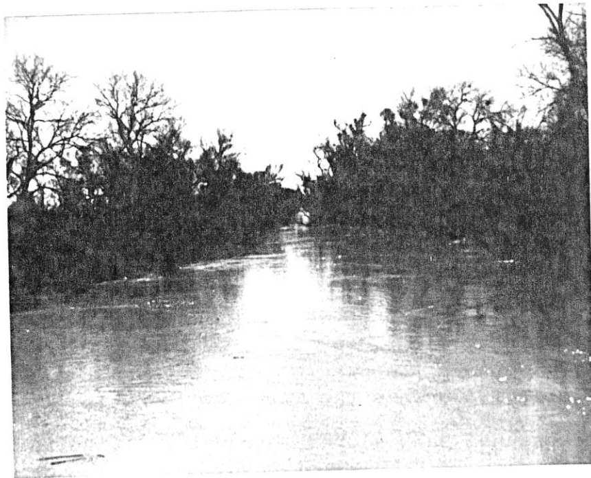
VEGATATION OVERGROWTH IN DRAIN LOOKING SOUTH FROM TULE ROAD BRIDGE
