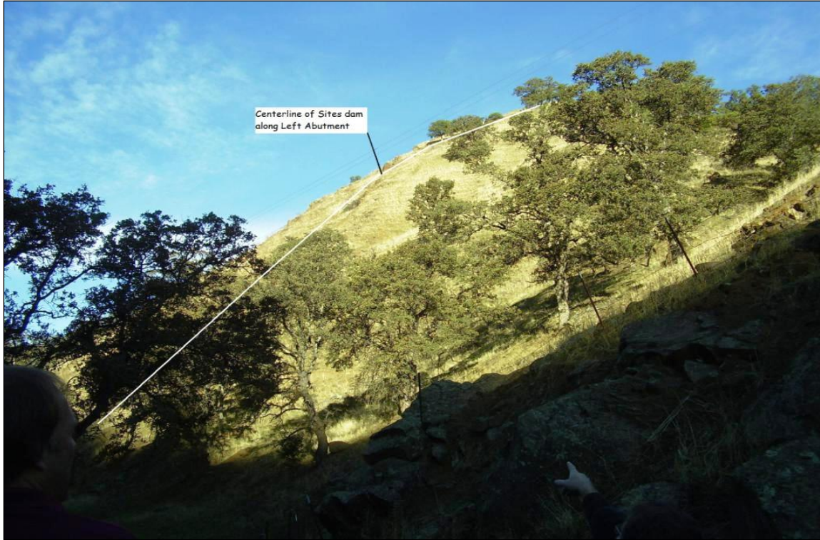
Photograph 1: Stone Corral Recreation Area showing centerline of Sites Dam along center abutment.
