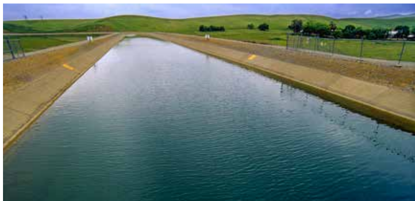
NODOS would take advantage of existing water facilities, including Tehama-Colusa Canal, as shown here.
