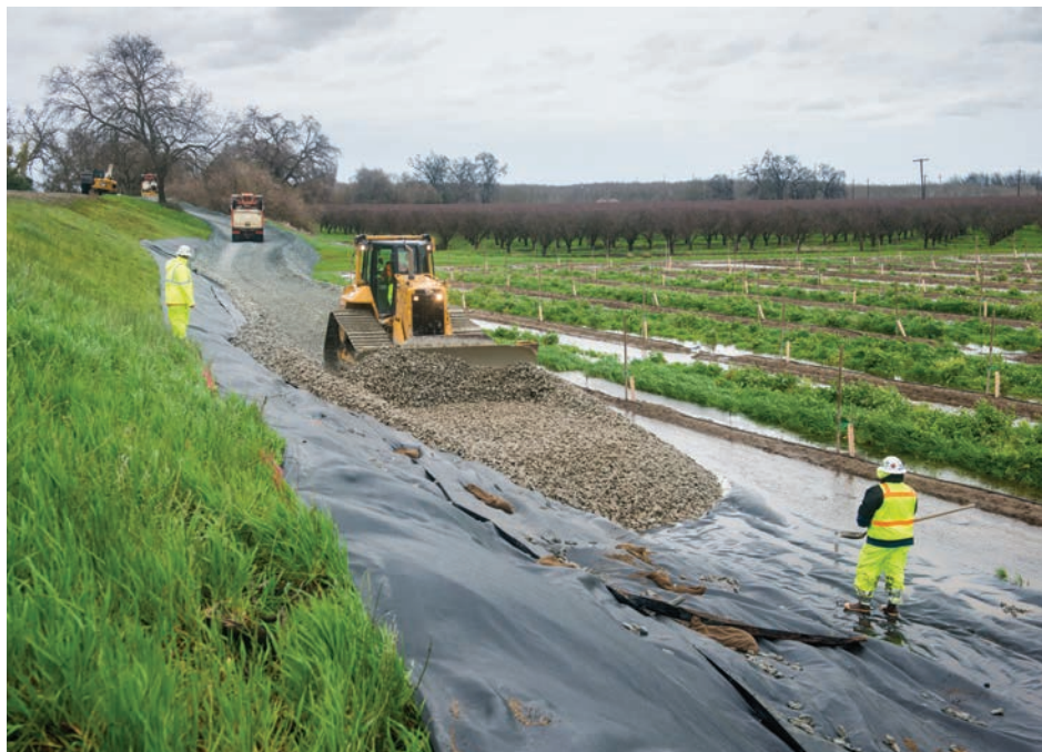
A Delta levee being repaired.
