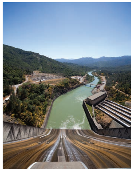
Shasta Dam operations affect salmon migration.
