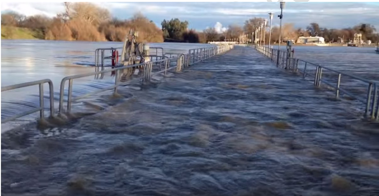
Figure 11-11. Streamflow Overtopping the Fish Screen Structure at Glenn-Colusa Irrigation District Hamilton City Pumping Plant, February 18, 2017.
